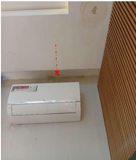
Pic showing the visible appearance of Pop discolouration due to water leakage from the Master bedroom terrace
