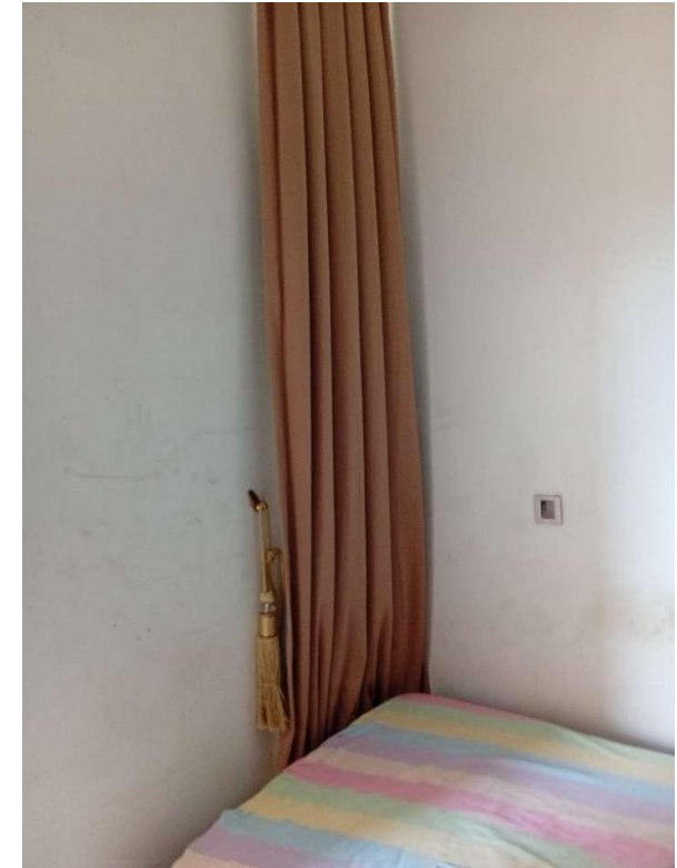
Pics showing a small window size, causing poor ventilation and poor natural lighting in the room.
