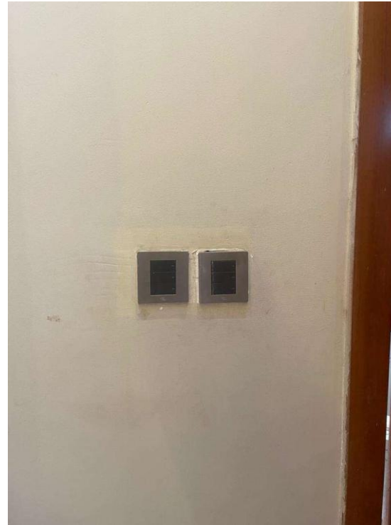
Picture showing aligned switches
