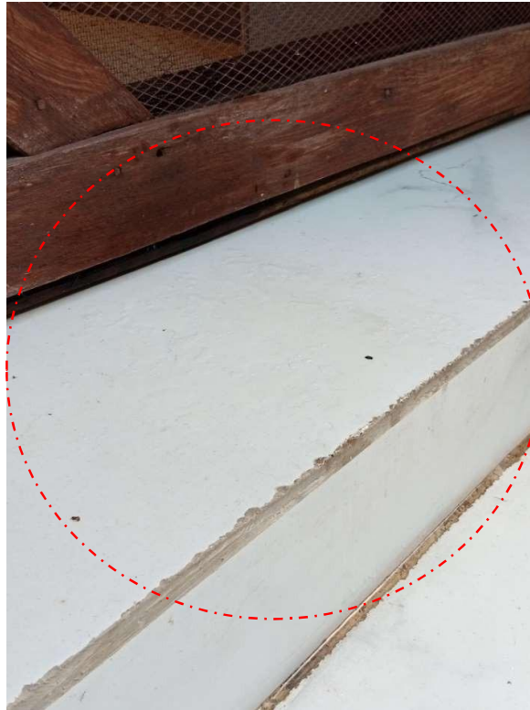
Pics showing water consistently dripping from the outdoor unit of the air conditioning system located near the kitchen exit door. This condition poses a potential slip and fall hazard.
